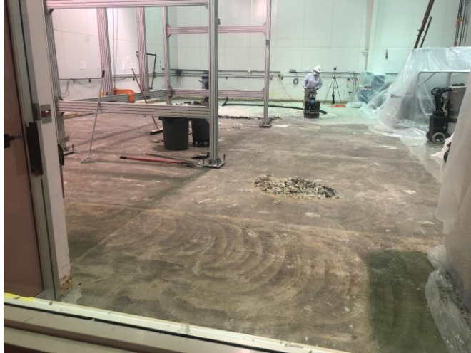
Day two progress of EEL cleanroom floor project
